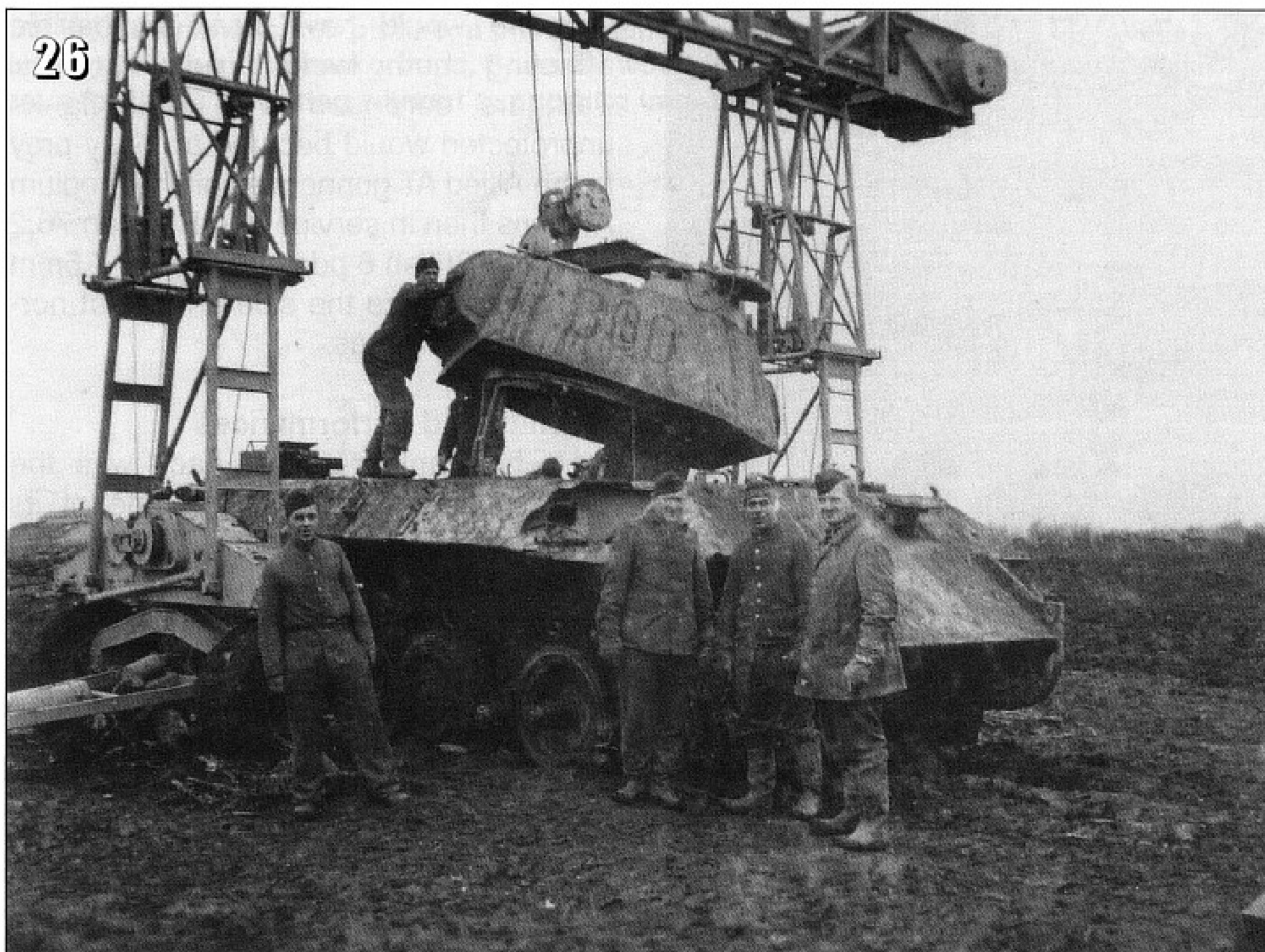
26- A picture is often worth a thousand words! Work being performed on a Panther Ausf. D in some very difficult conditions, during the winter of 1944. This tank hull looks badly damaged by AT weapons and it is probably being disassembled to salvage any useful parts. The lack of spares often led to cannibalisation of inefficient tanks to maintain the readiness levels of the armoured units. (Anderson)
